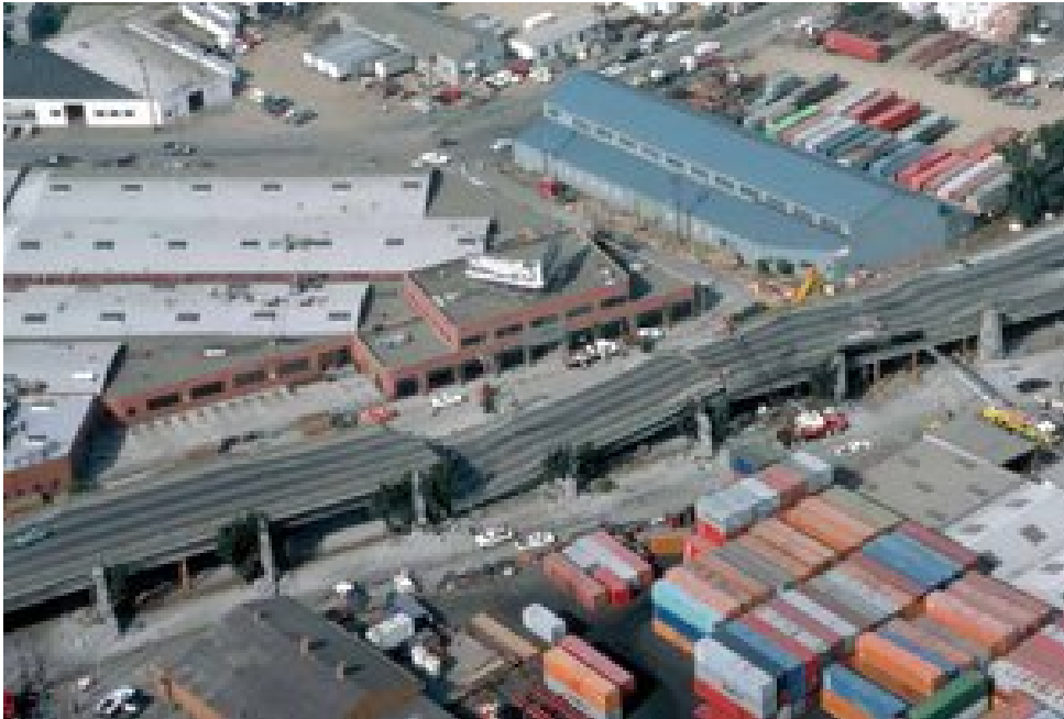
Loma Prieta (October 17, 1989) Case study of highway failure
